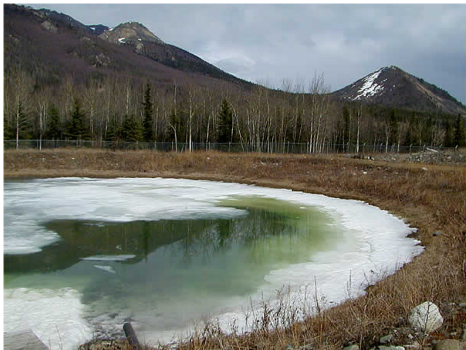
Fig. 6.6 Example of a facultative lagoon for waste water treatment near Denali National Park and Preserve. Note the ice cover and spring thaw.
