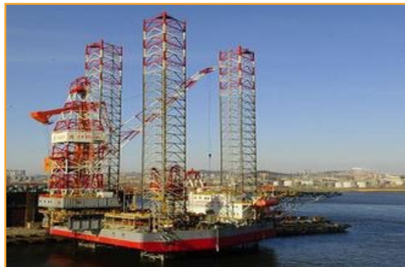
Jack up drilling platform above 120 meter water depth
