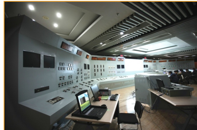
Sodium cold test fast reactor simulation
