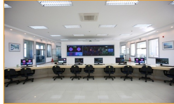
Independent development of digital simulation system for nuclear power station
